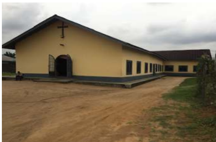
Plate 3c: The first church building standing completed.
