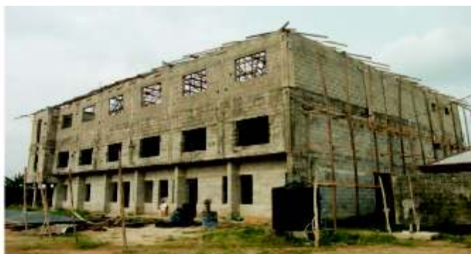
Plate 3h: Showing Church of the Nativity Parish hall under construction
